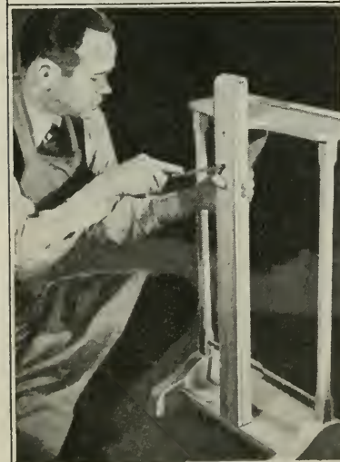
The bracket is screwed in place
